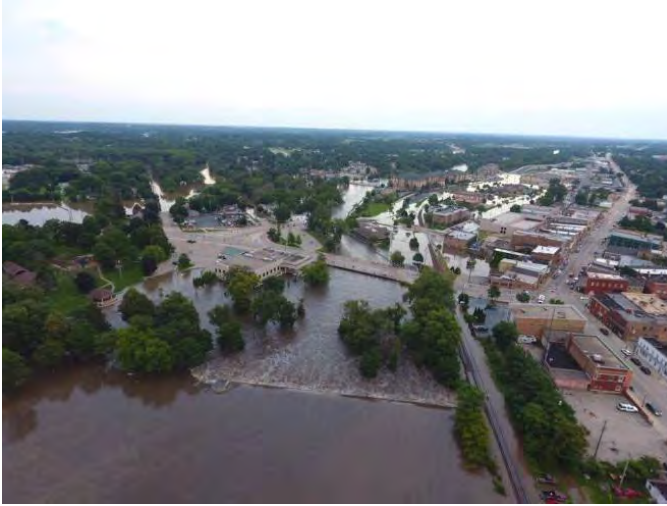
Figure 3.1 July 12, 2017, Flooding: Fox River in the City of Burlington
