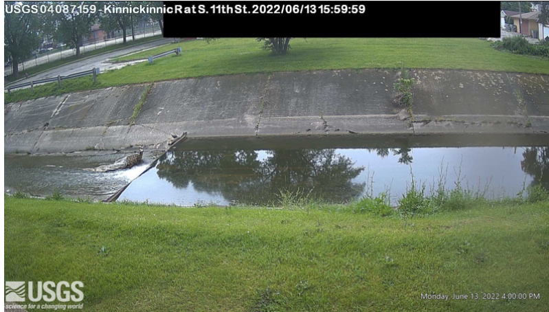
Figure 5.5 Milwaukee Metropolitan Sewerage District Watercourse Corridor Study: Real-Time Imaging Data Collection on Kinnickinnic River Mainstem at S.11th Street: 2022
