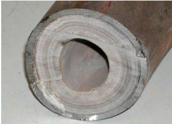
Figure: 5.1 Scale Build-up in a Water Pipe
