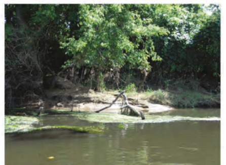
22 - DRAIN TILE OUTLET DEPOSITION
