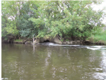
2 - WASTEWATER TREATMENT PLANT OUTLET
