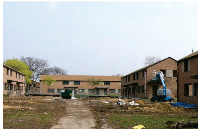
Westlawn Demolition and Renovations Underway
