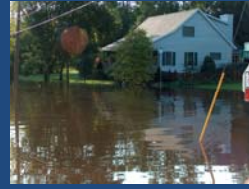
Flooding and Stormwater Drainage Problems
